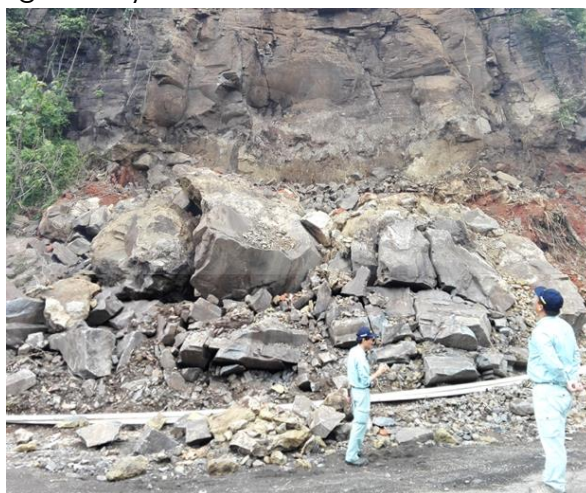
Figure 6.8 Collapse of rocks induced by rains on the national route RN-15. June 2018. (MOP El Salvador)
