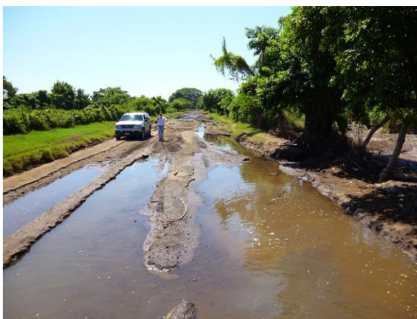
Figure 6.4 Flood due to channel change due to storm 12E, Usulután Salinas Sisiguayo, El Salvador 2012 (MOP El Salvador)
