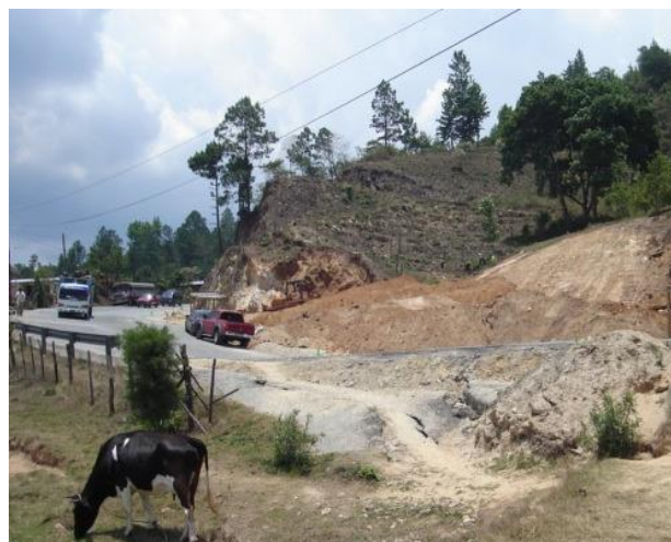
Figure 2.4 Traction cracks caused by filtration and hydrostatic pressure. Taken on road CA-14 Guatemala
