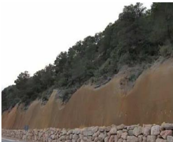
Figure 2.3 Drain concentration in a road cutting
